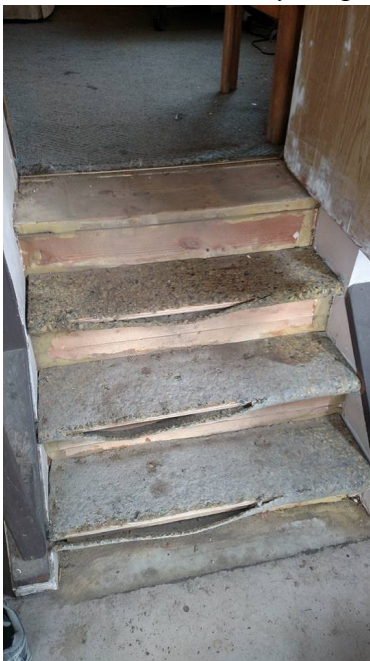
Removing the carpet from the stairs.
