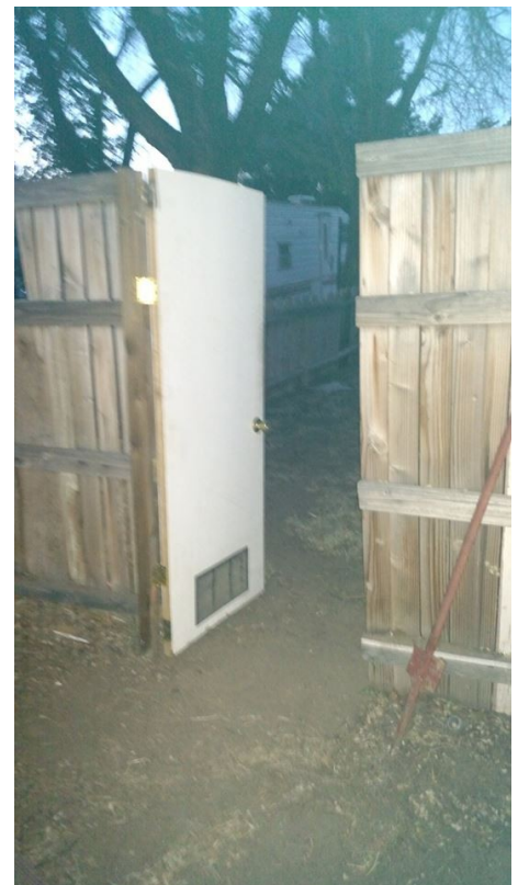
Door installed (photo taken at night).
