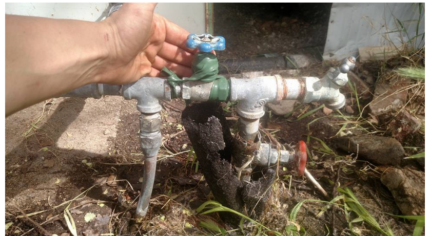
After mending the pipeline using plumber's tape from L & M Lumber.
