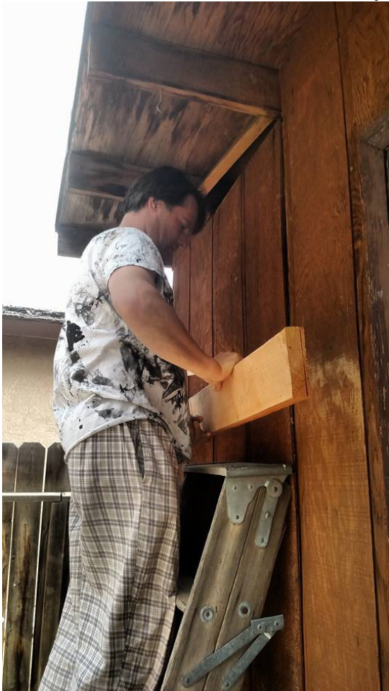
Friend Daniel Wulff, a skilled builder, helped to fix the hole.
