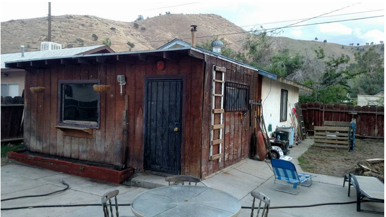
Got window replaced. Hanging planters gifted from Renee and Adam Forker . Glass table in foreground from neighbor Mark . Ladder built by us to access the rooftop.
