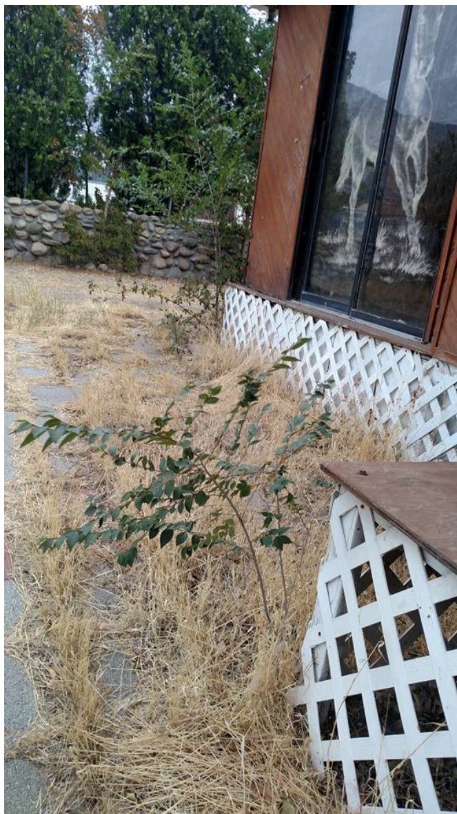
Notice that the shrubs surrounding the house are "aimed" inward, with roots headed toward water pipelines.
