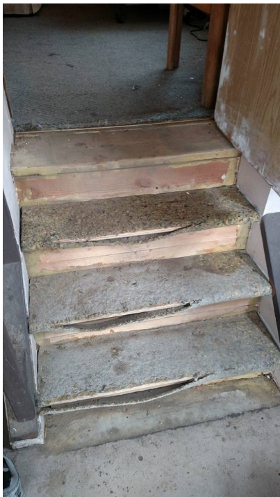
Removing carpet from the stairs.
