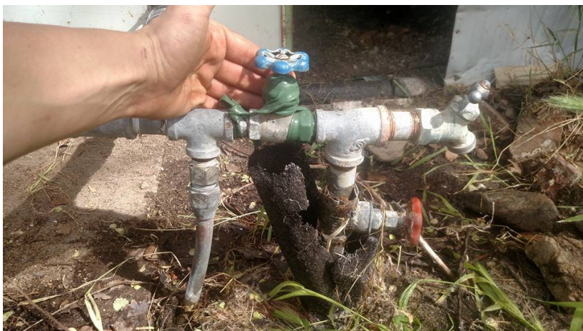
After mending the pipeline using plumber's tape from L & M Lumber.
