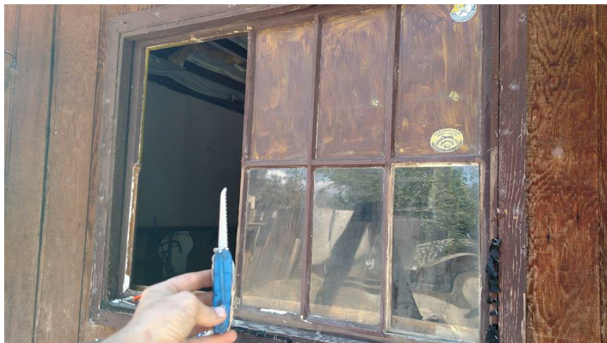
Cutting out the window with a Swiss Army knife.
