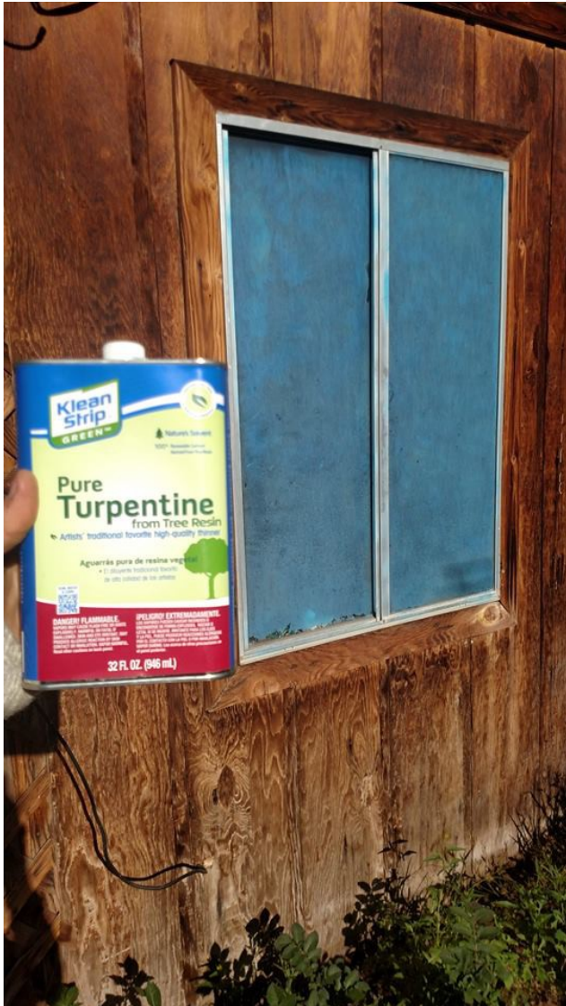
4-8-2016: About to scrape the paint off, then clean it with turpentine.
