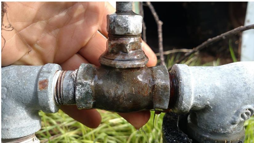
The main line to the water supply before we mended it.
