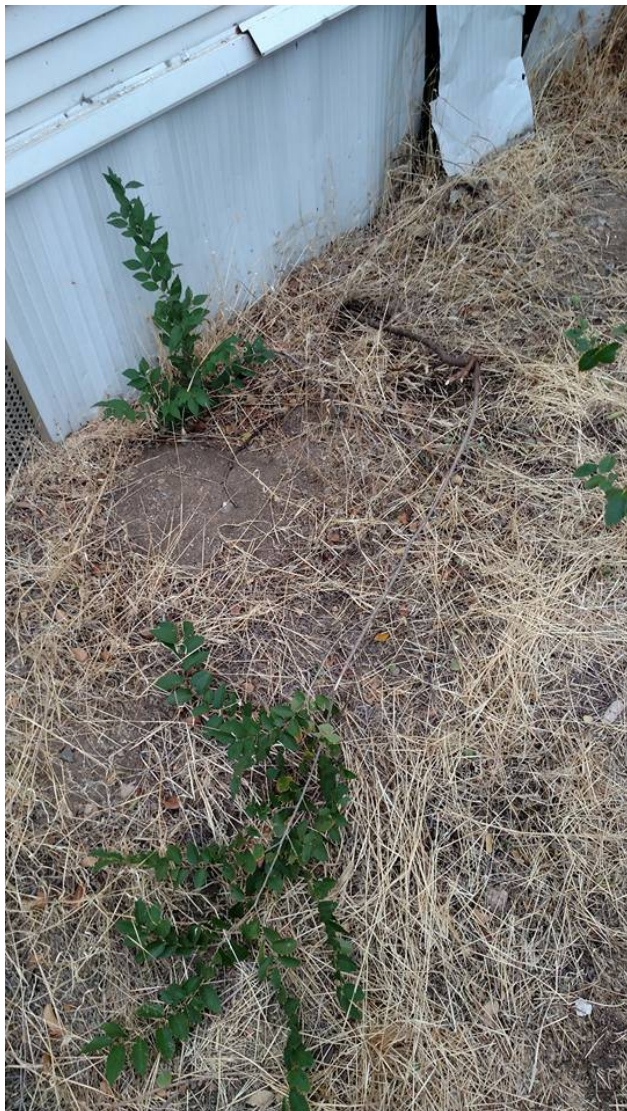
Removed invasive shrubs from all 4 sides of the property; notice the long root aimed directly under the house - see page 7.
