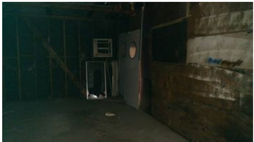
In adjacent room beyond the meat locker doors, looking back toward them. Broken glass scattered across the floor.
