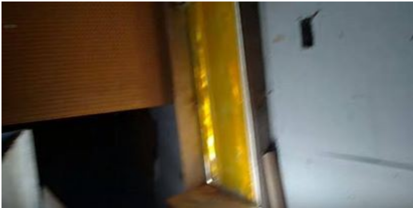
Looking up and to the right from the previous photo – wooden pegboard hanging from the ceiling, window painted yellow.
