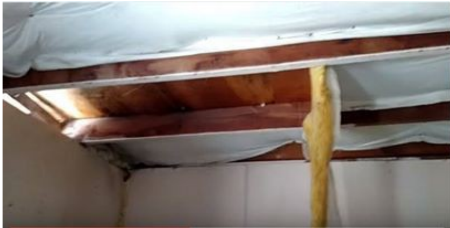
Insulation hanging from ceiling, hole in wall.
