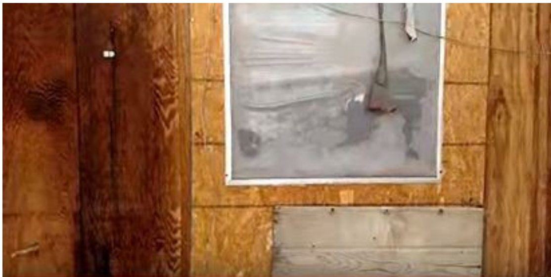
Facing window directly south of walnut tree.
