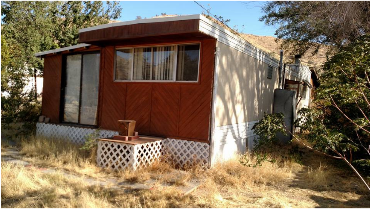
Dried grasses imposed a fire hazard to the property and neighborhood.
