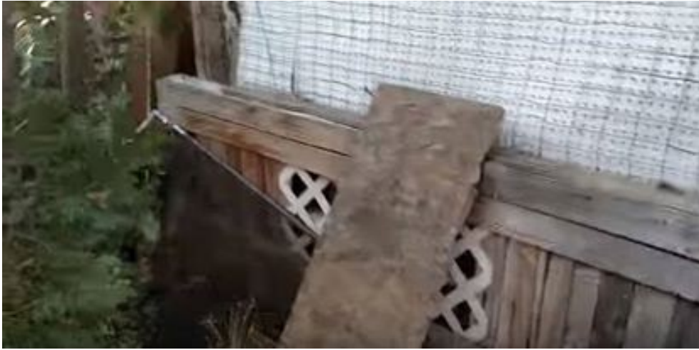
Looking slightly westward from previous photo – a wooden contraption attached to house is surrounded by debris.
