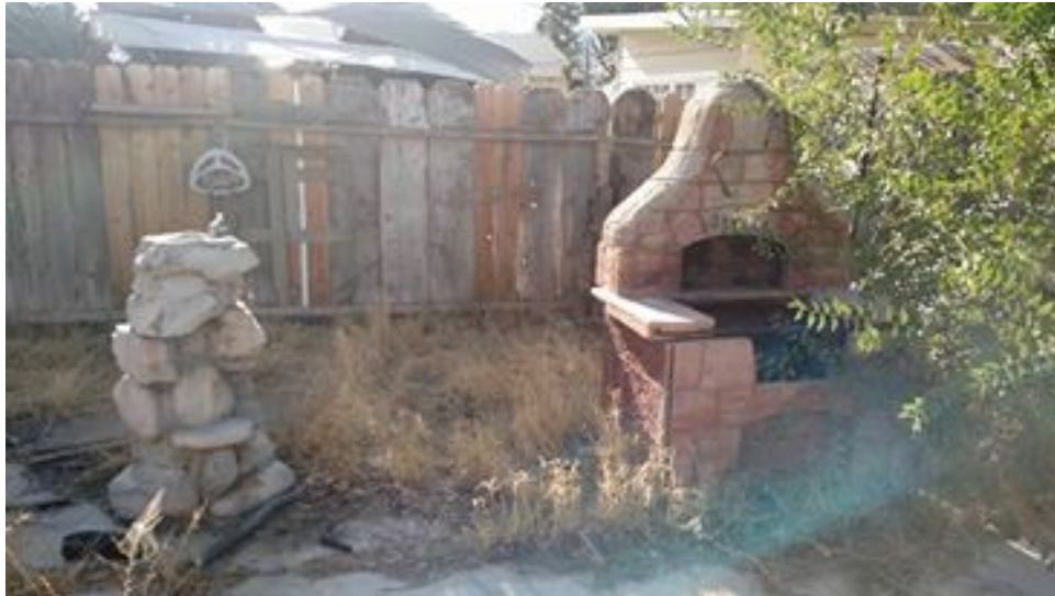
Dried grasses imposed a fire hazard to the neighbor's property and fence.
