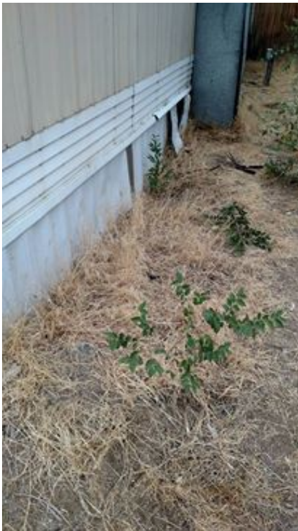
Root systems of invasive shrubs on west side of house grew toward waterlines beneath the house – see pages 50 and 51.
