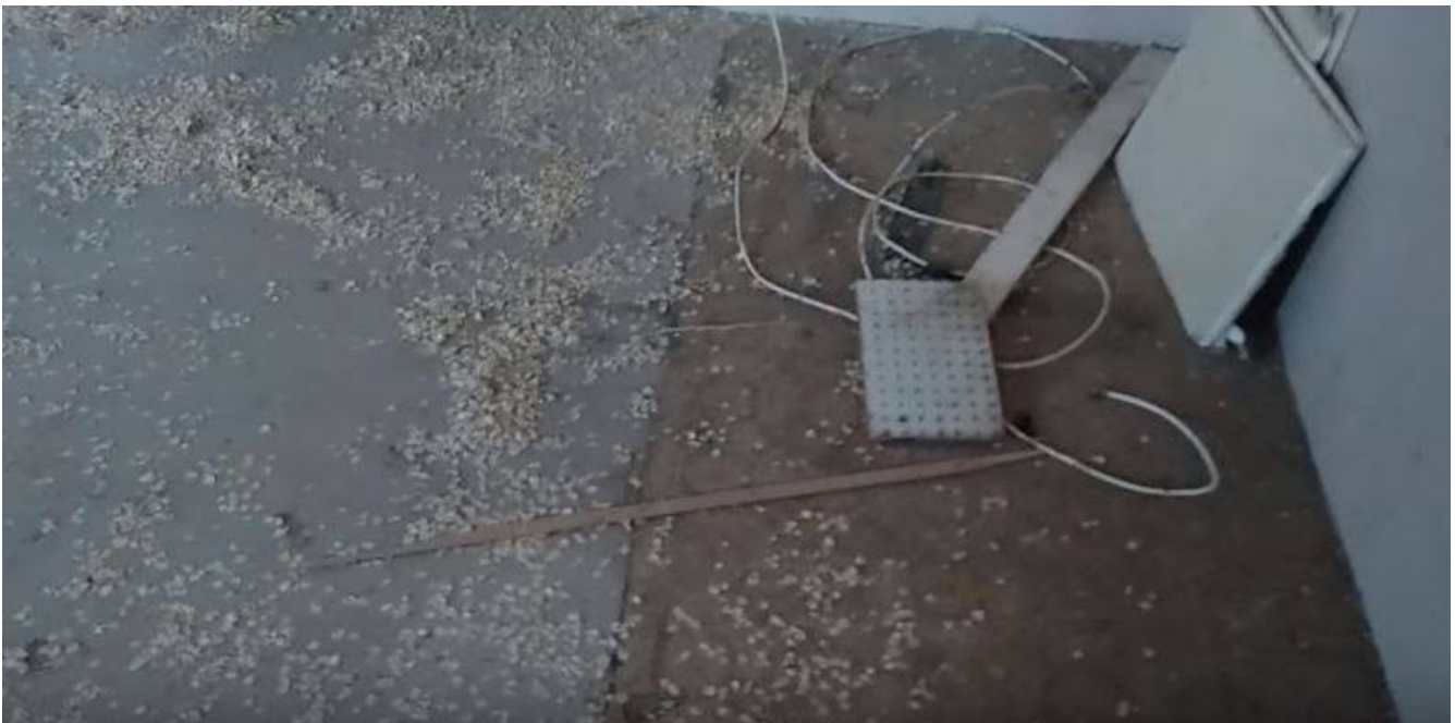
Floor covered with insulation and debris.
