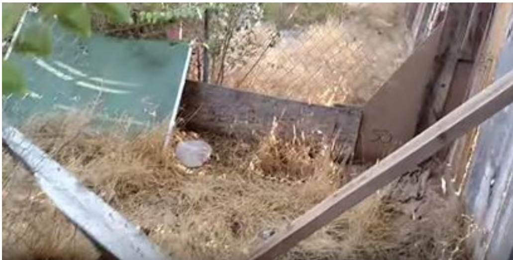
Stepping to the right from previous photo; debris.
