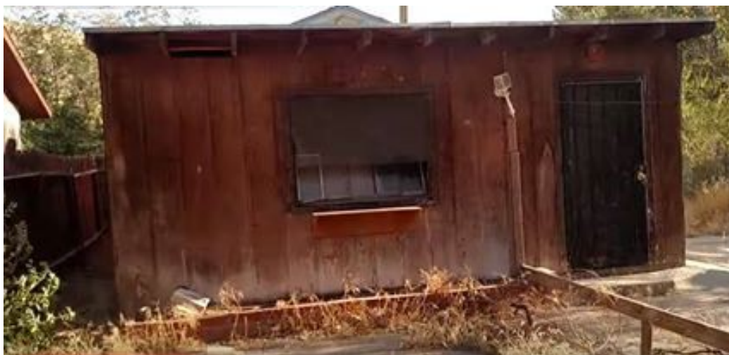
Front of rear building.
