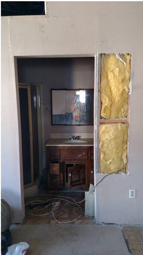
Looking into bathroom (after we swept the floor).
