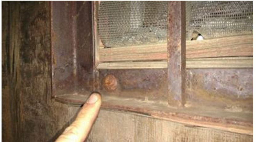
Closeup of barred window on left from above photo – glass window shattered.
