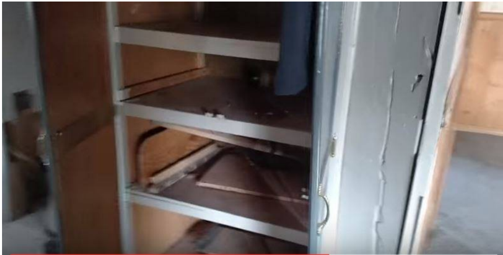
Turning to the right (east) from previous photo. Cupboards covered in dust.
