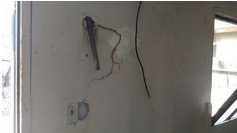
On left side of the top photo on previous page – wooden handle bashed into the wall as discovered.
