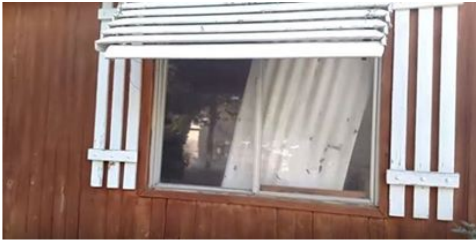
First window on the right – metal panel leaning against glass.
