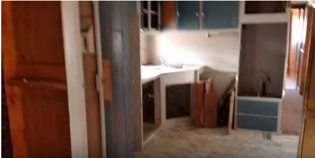
Stepping forward from previous photo, into the kitchen. Appliances missing.
