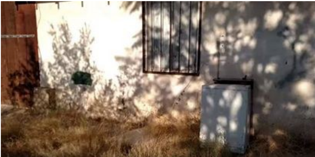
Facing west side of rear building – old broken washing machine sitting outside.
