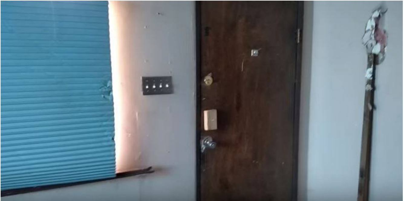
A 2" x 4" piece of lumber was bashed into the west wall.
