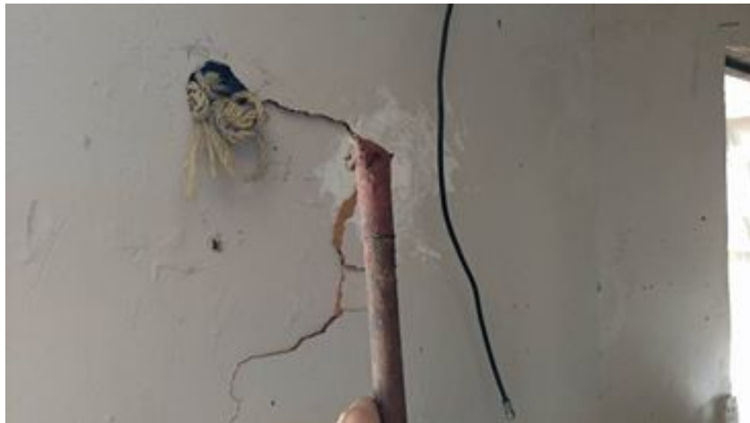
Pulling the handle from the wall, showing how previous occupants left the building.
