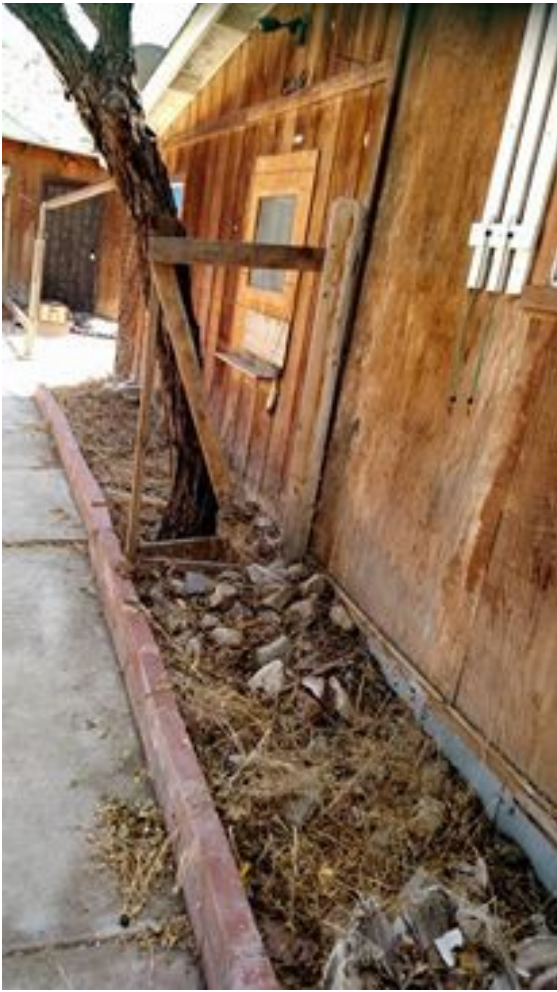
East side of house, brick garden filled with rocks and trash. Wooden contraption nailed to the walnut tree.
