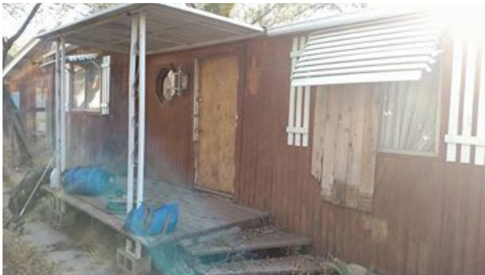
Front porch, boarded up, paint chipped.
