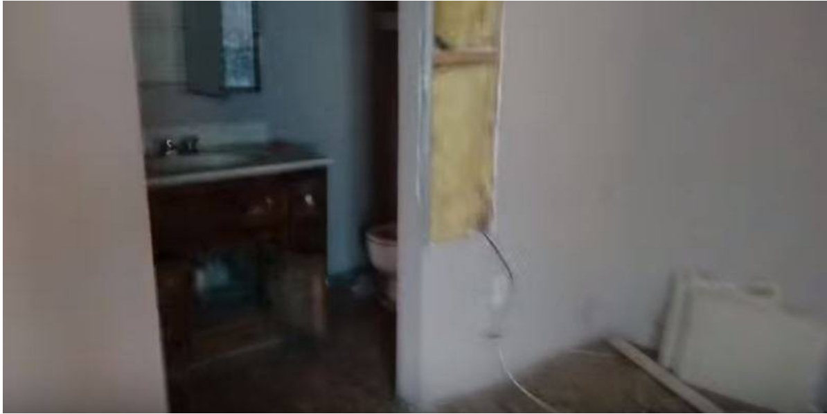
Facing northwest in master bedroom. A chunk of wall is missing, and a cord is pulled out from it is strewn across into the room .
