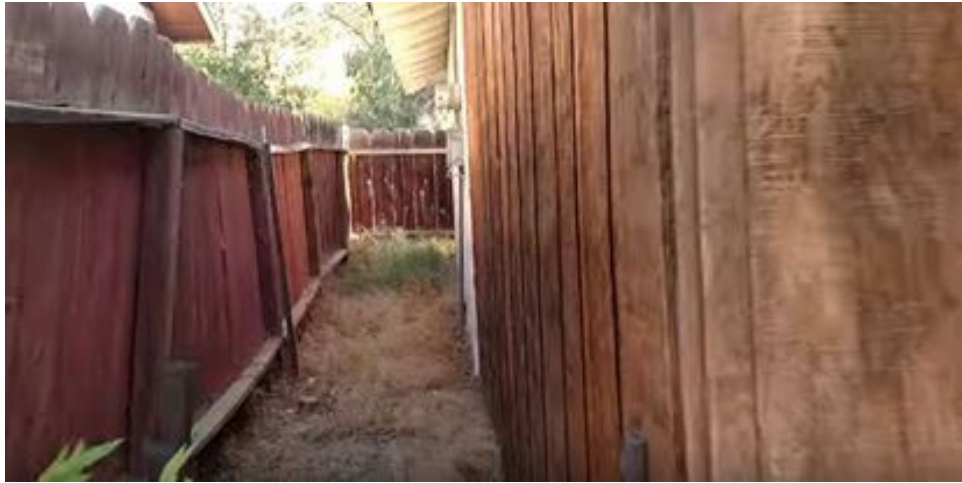
Behind rear building at south side of property, facing west. Dry grasses threaten wood building and fence.
