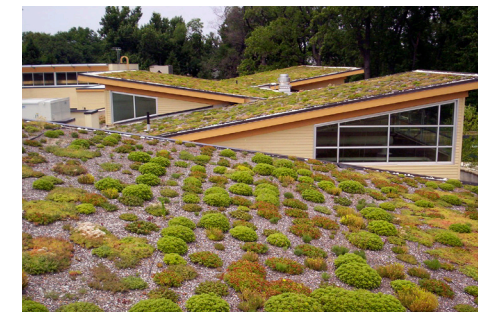
The vegetated roof at Walter Reed Community Center in Arlington, Virginia. Photo: Arlington County
