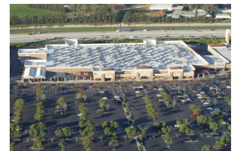
The Walmart and Sam’s Club in Chino, CA, are both equipped with white roofs and solar panels to help Walmart reach its goal of being supplied by 100 percent renewable energy. Photo: Walmart Stores
