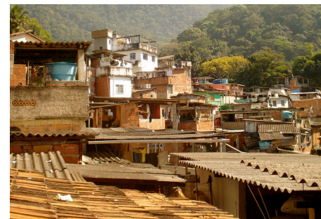
Corrugated metal roofs in Rio de Janeiro. Photo: whl.travel
