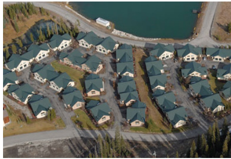
Cool colored metal roofs. Photo: Custom Bilt Metals
