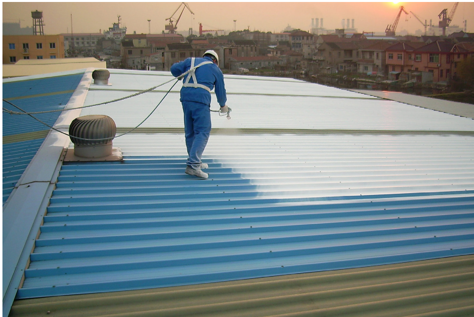
Applying white coating to a roof in China. Photo: United Coatings
