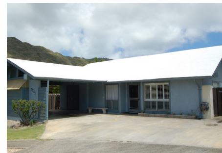
A cool roof in Hawaii. Photo: Mikenan1
