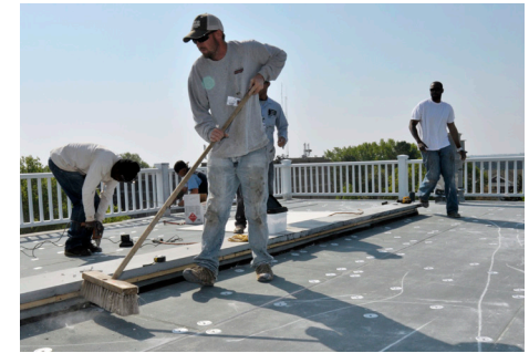
Workers install a white roof on a museum building at University of Central Arkansas. Photo: UCentralArkansas
