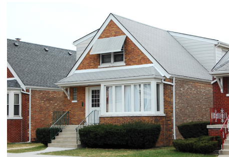
A steep-sloped single family home with asphalt roof shingles in the U.S. Photo: Eric Allix Rogers
