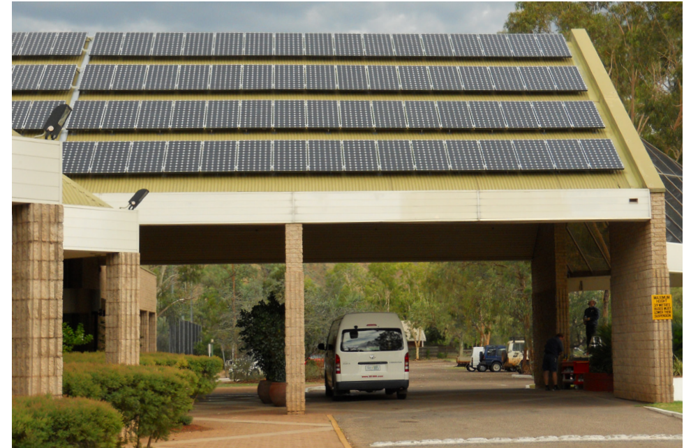
A solar PV roof in Australia. Photo: Neal Jennings
